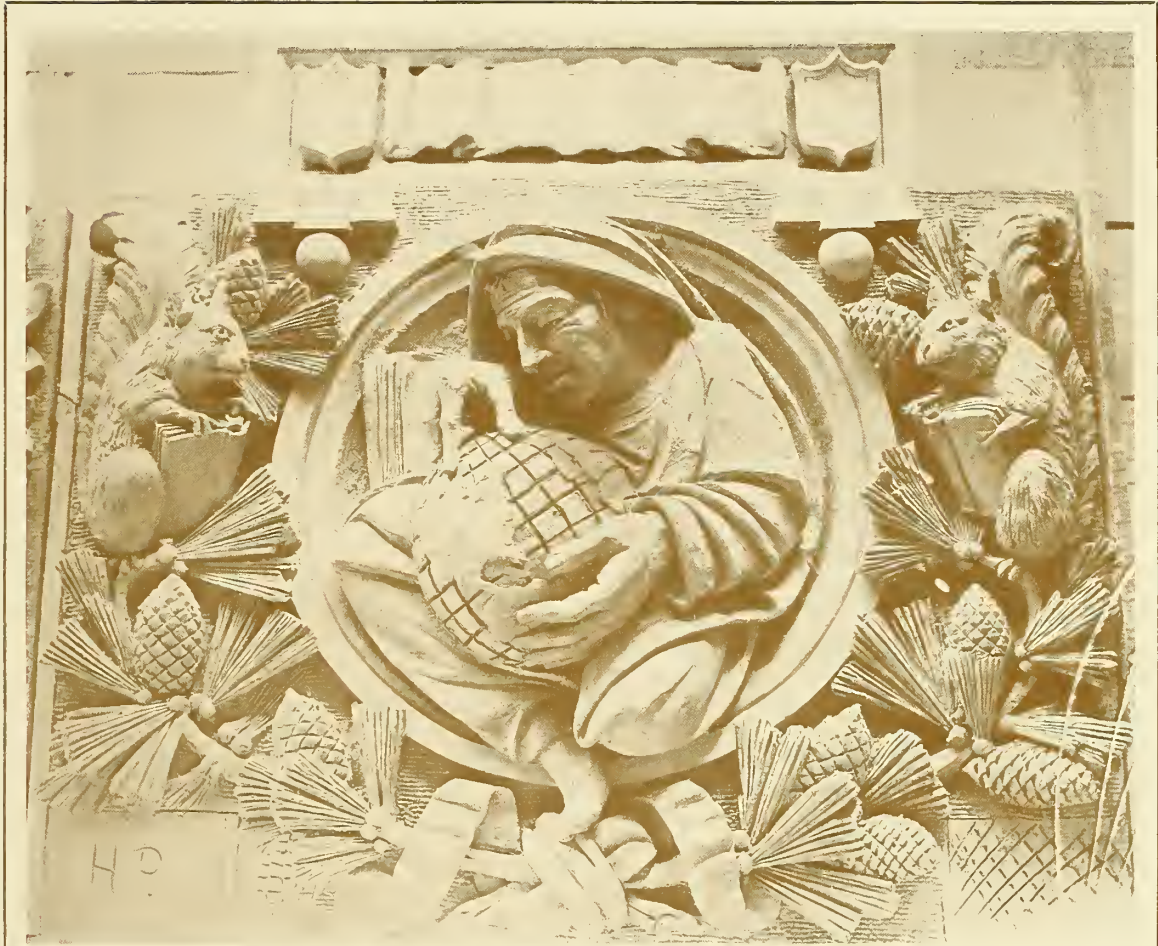
One of several panels made for the WM. F. HARRITY SCHOOL, 56th and Christian Sts., Philadelphia, Pa.
